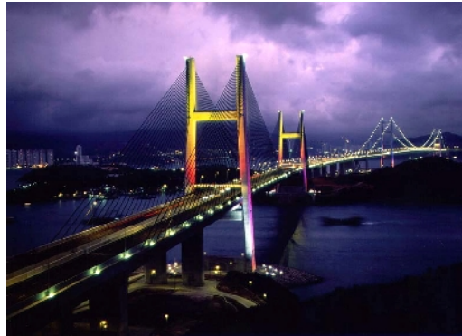
Tsing Ma Bridge, HK (+300 channels)
