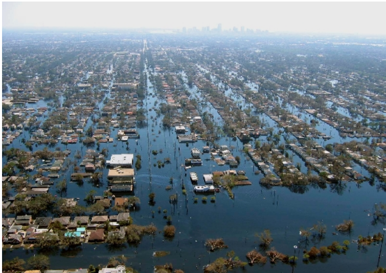
Hurricane Katrina (2005) Failure of levees lead to cascading failures
