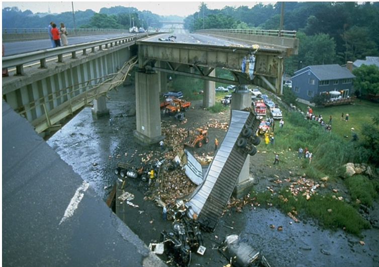
I-95 Overpass Collapse (1983) Corrosion beneath pin hanger leads to fatigue
