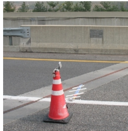
Installed PVDF strips
