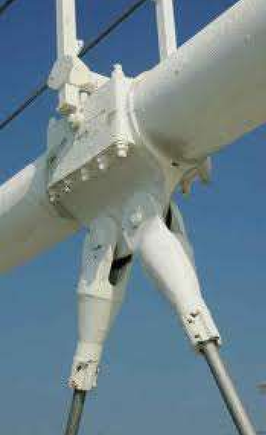
Pin plate connection
