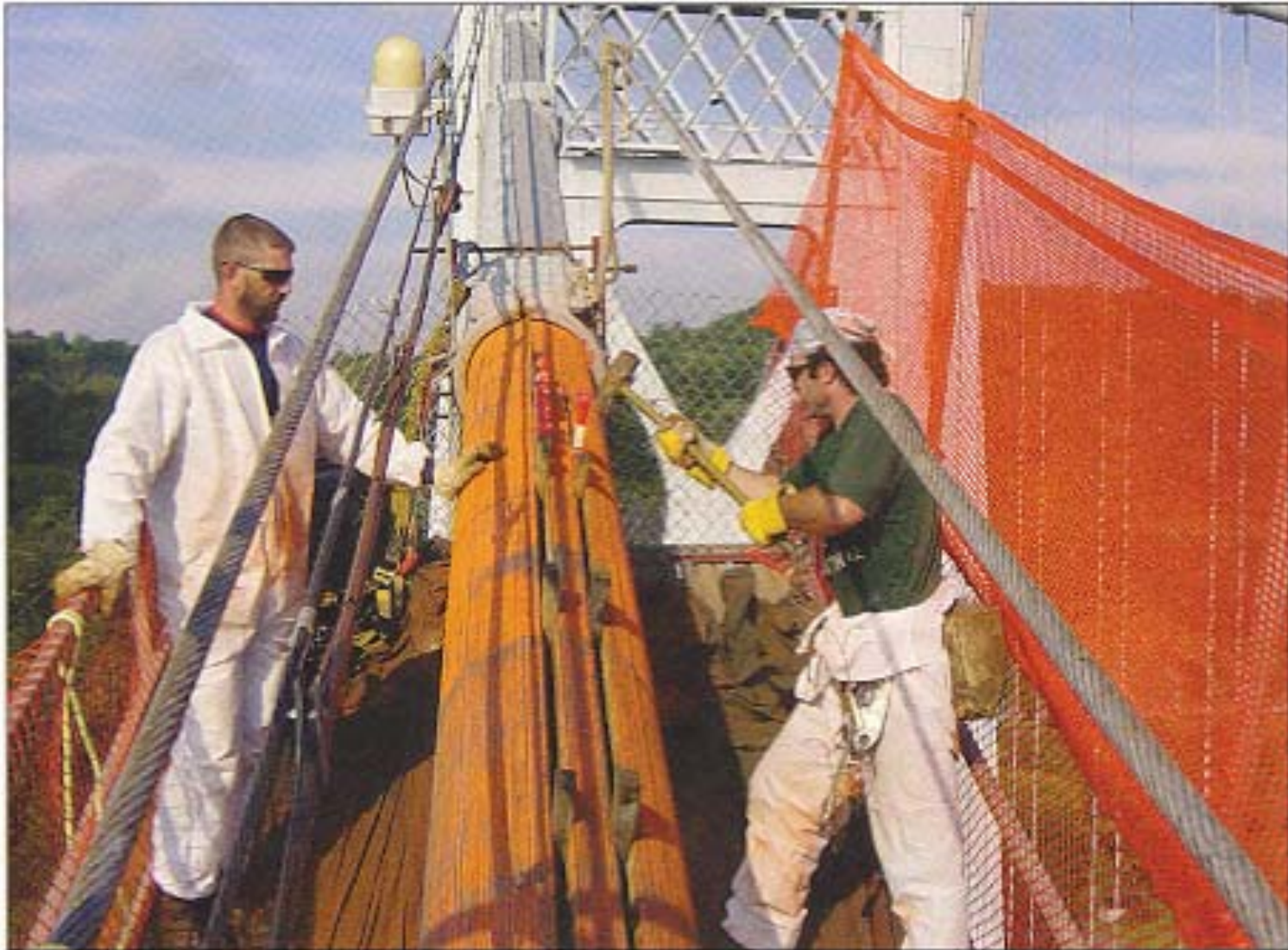
▲ Cable Close-Up. Bridge crews insert wedges to open up a cable in Mid-Hudson River Bridge.
