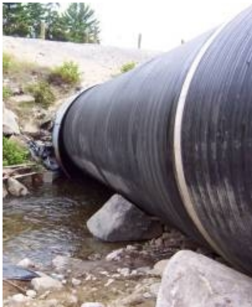
Culvert lining, East ON
