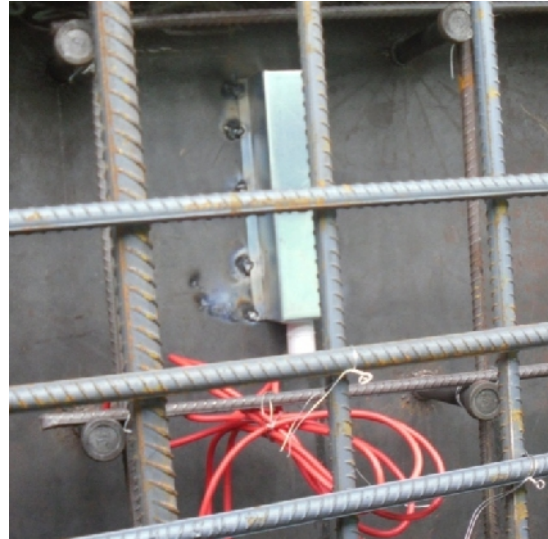
Strain sensors (vibrating wires) installed on the embedded steel column of one mega column – to measure the strain of the steel
