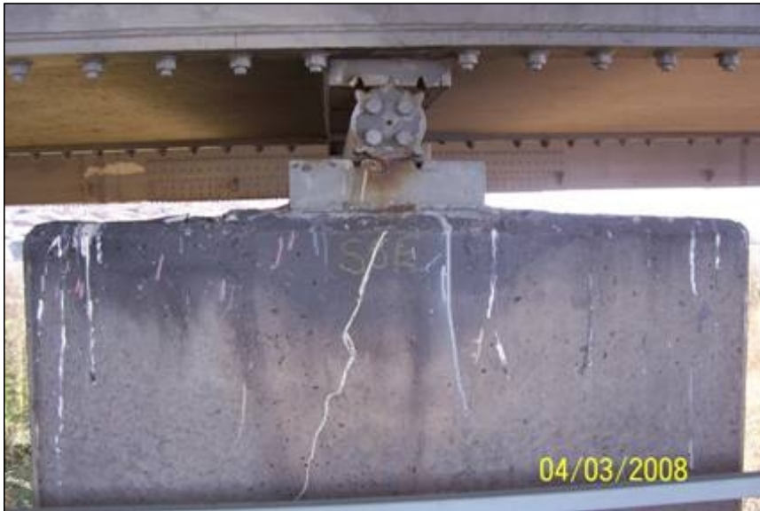
Typical Steel Roller Bearing
