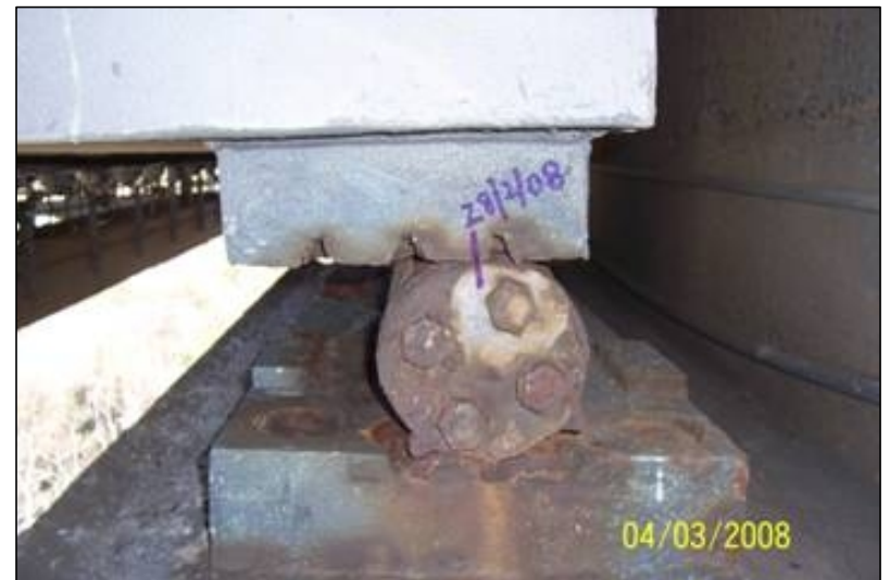
Roller bearing at north side tower
