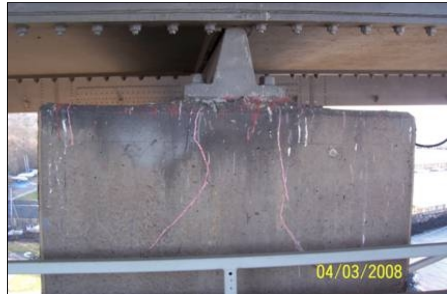
Typical Steel Rocker Bearing
