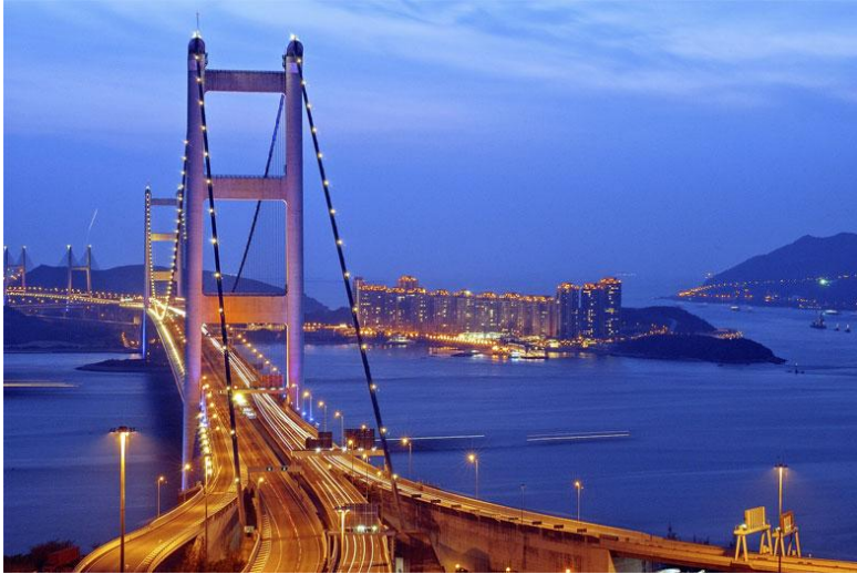
Tsing Ma bridge, Hong Kong
