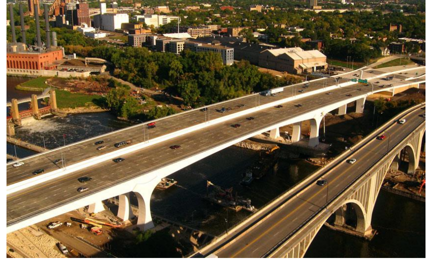
St. Anthony falls bridge, Minnesota
