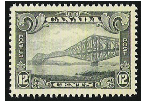
2 nd Quebec bridge, 1916
